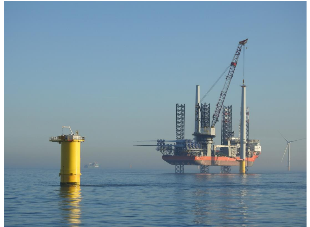
The Pacific Osprey completing turbine installation at Triton Knoll.
