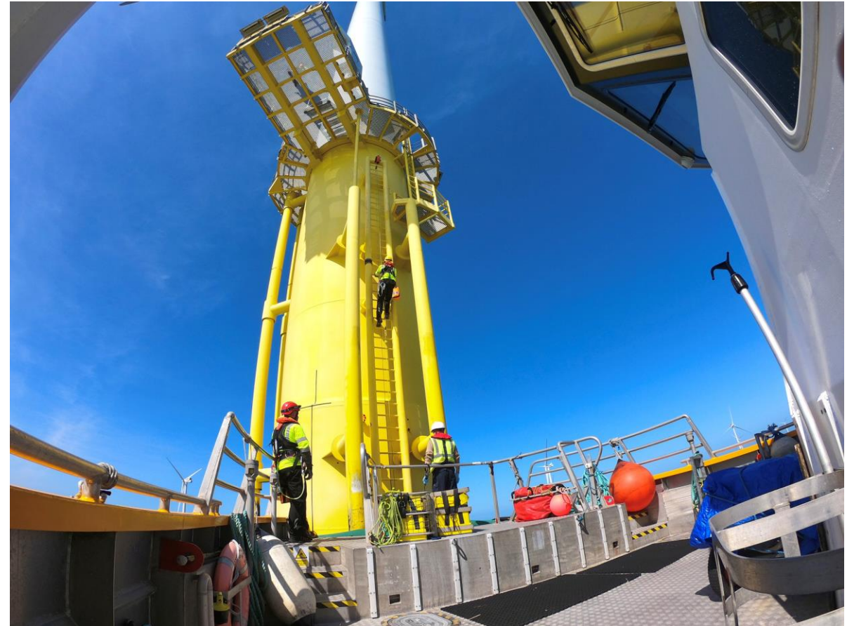
Maintenance underway at Humber Gateway Offshore Wind Farm
