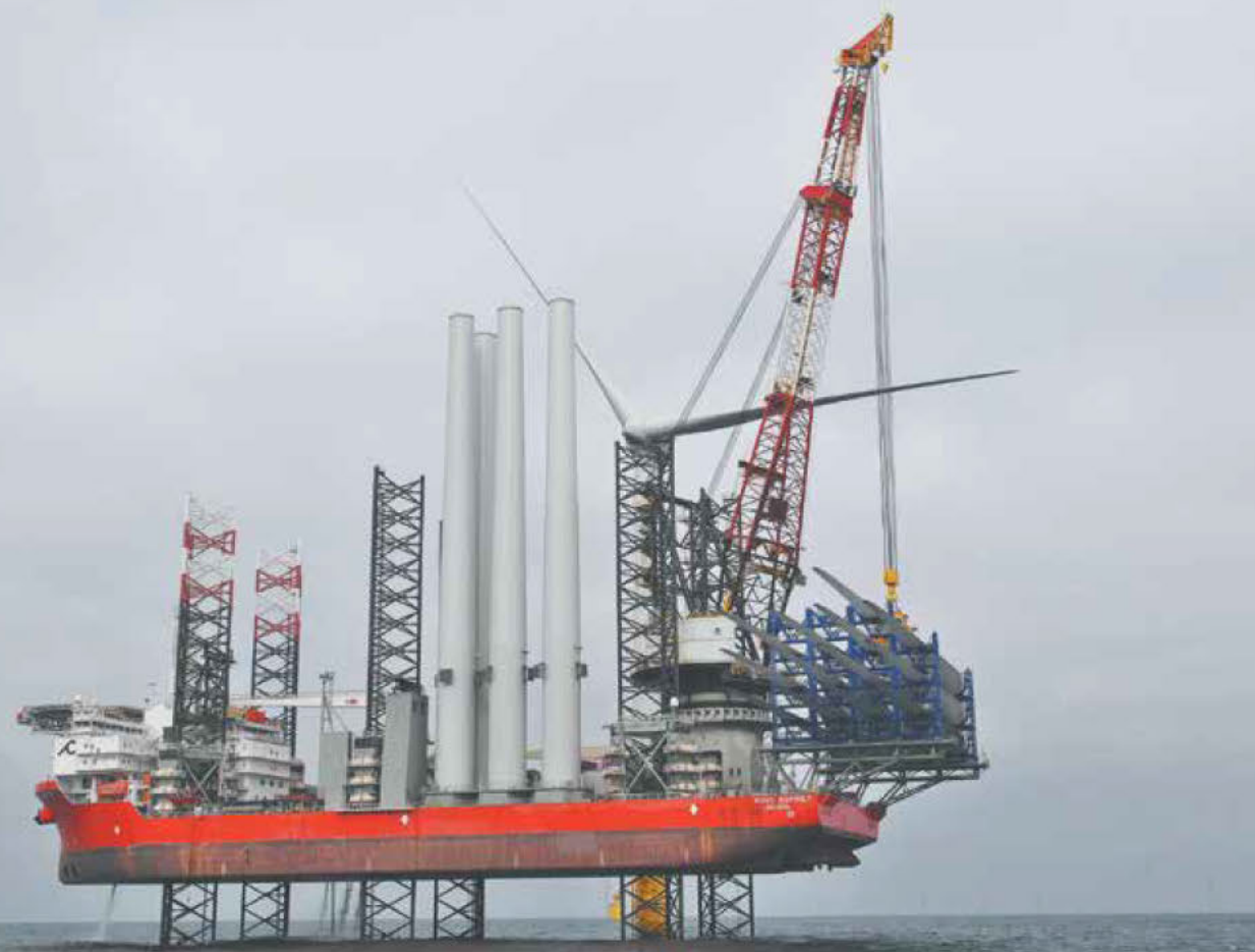
Turbine installation at Triton Knoll Offshore Wind Farm
